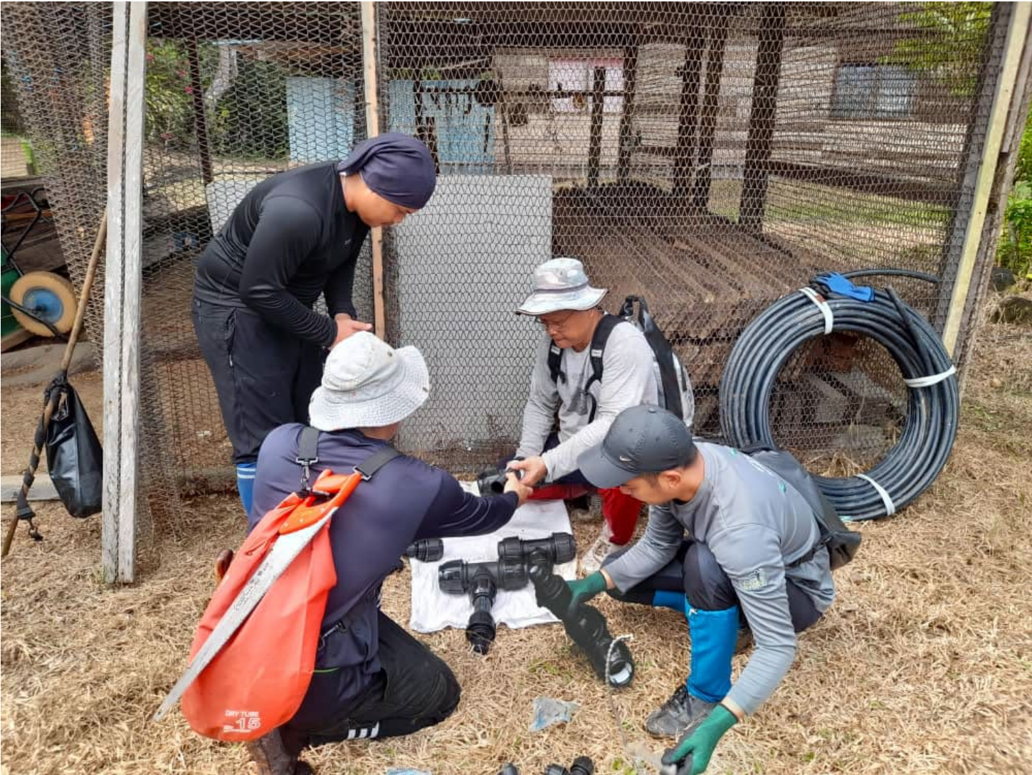
Project: Gravity Feed System at Long Kerong, Upper Baram
